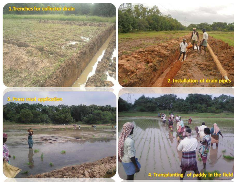
Plate 1. Constuction of control drainage system
