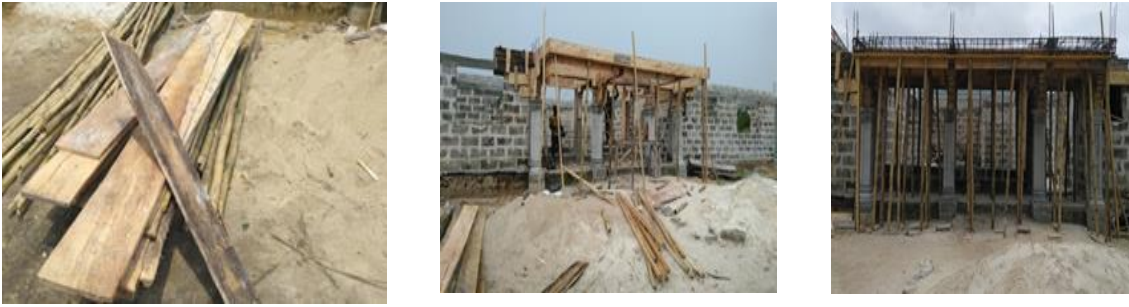
Fig. 2. Rubberwood boards and props as construction materials; Ozoro Delta State, Nigeria
